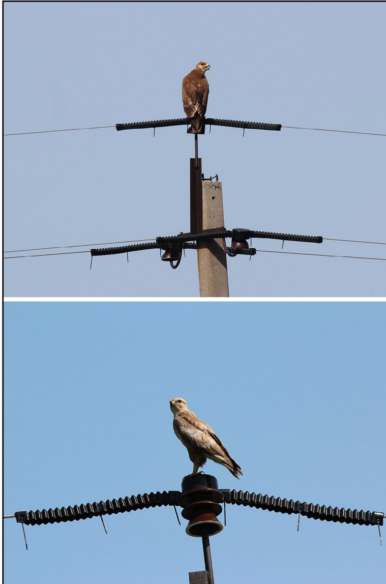
Steppe Eagle (Aquila nipalensis) and Common Buzzard (Buteo buteo) on power poles with bird-protective covers from the Eko-NIOKR company.
