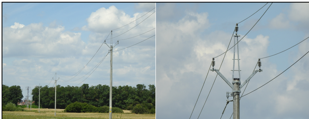
Fig. 3. For newly constructed lines, crossarms with side arms angled upwards are often used. This is both a long-lasting and a very effective measure. Photos from Raptor Protection of Slovakia.
