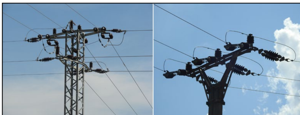
Fig. 1. Branch supports (left) and poles with jumpers above the insulators (right) pose the highest risk of electrocution in Slovakia. Photos from Raptor Protection of Slovakia.
