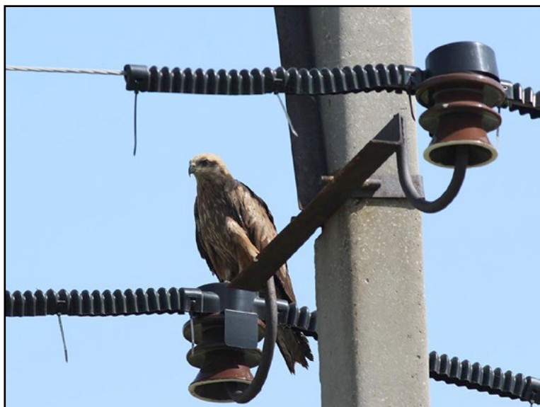
Black Kite (Milvus migrans) on power pole with bird-protective covers from the Eko-NIOKR company.
