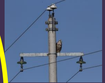
Suspended Insulators
