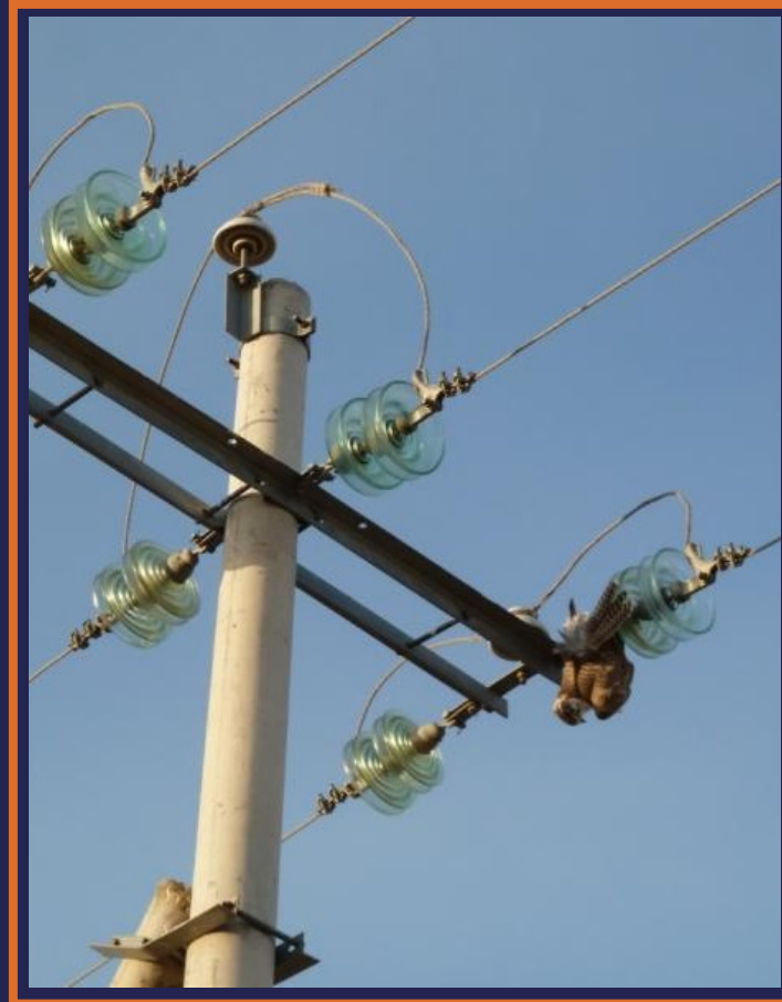
Galvanized steel supports
